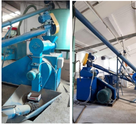
Figure 5. Pellet press – Pellet factory – INO-MAT project
